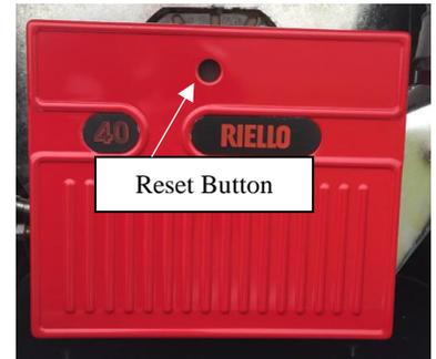
Figure 32 - Burner Reset Button
